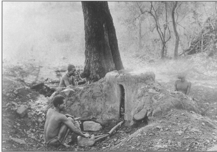
'Makaties iron foundry ... east of the Spelonken'. This remarkable photograph, taken in 1888 by H. Gros, shows a typical Venda iron-smelting furnace in operation. The operators are each using two bellows made of hide. Straightened antelope horns channel the air blast through three clay tuyères to the charge in the furnace (Africana Library, Johannesburg)
