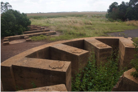
Circular foundations of a roaster
