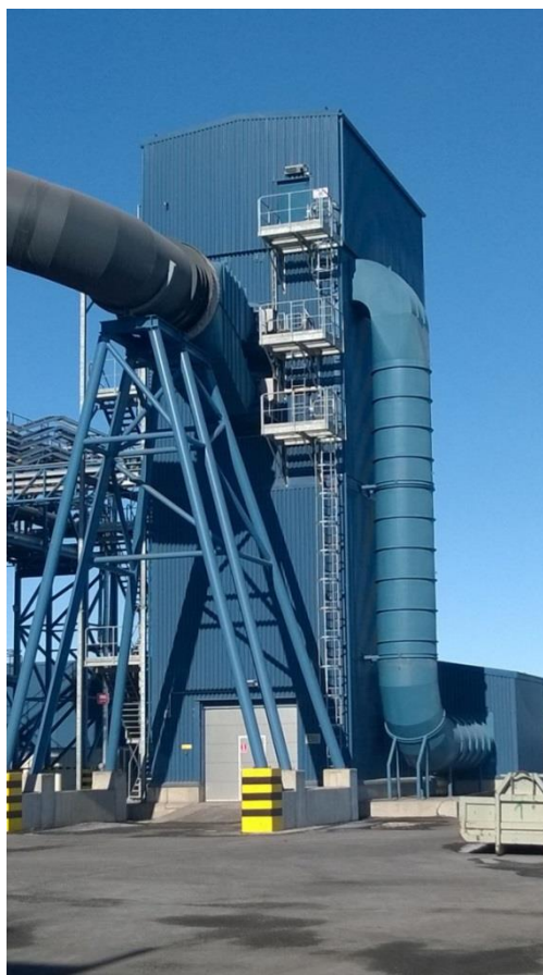
Figure 4. Bag filter unit for SAF3 tapping area fumes handling
