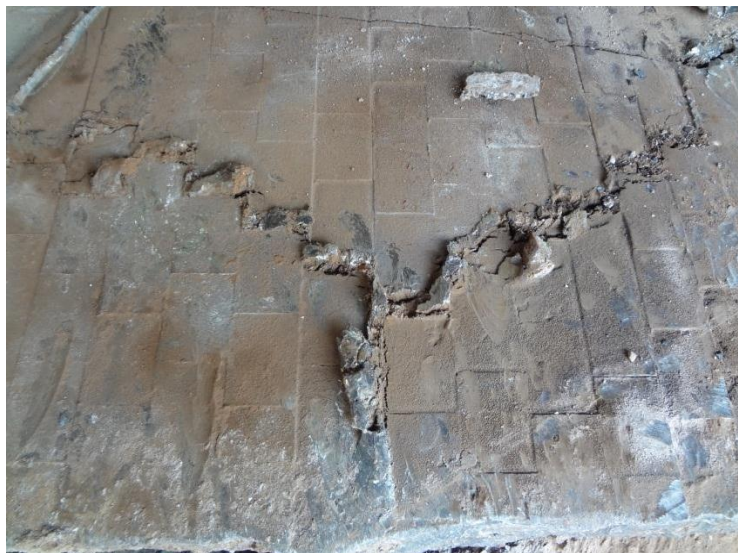
Figure 4: Onça Puma Hearth During Demolition
