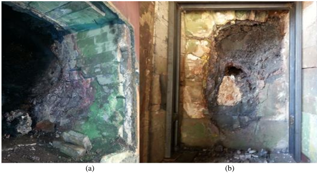
Figure 4 – (a) Tapping hole lining maintenance, Vargön Alloys AB ,Sweden (b) Tapping hole lining maintenance, Eti Krom Inc., Turkey
